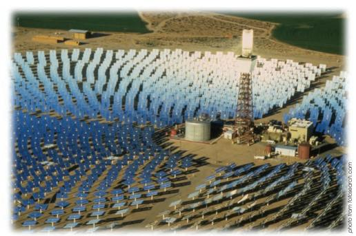
A solar power plant in the USA. It uses mirrors to focus sunlight onto a central tower. This is called a thermal solar power plant as it uses heat to change water into steam. The steam drives the generator.
