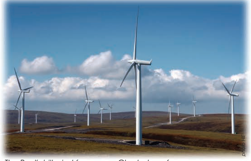
The Paul's Hill wind farm, near Charleston of Abellour, Moray.
