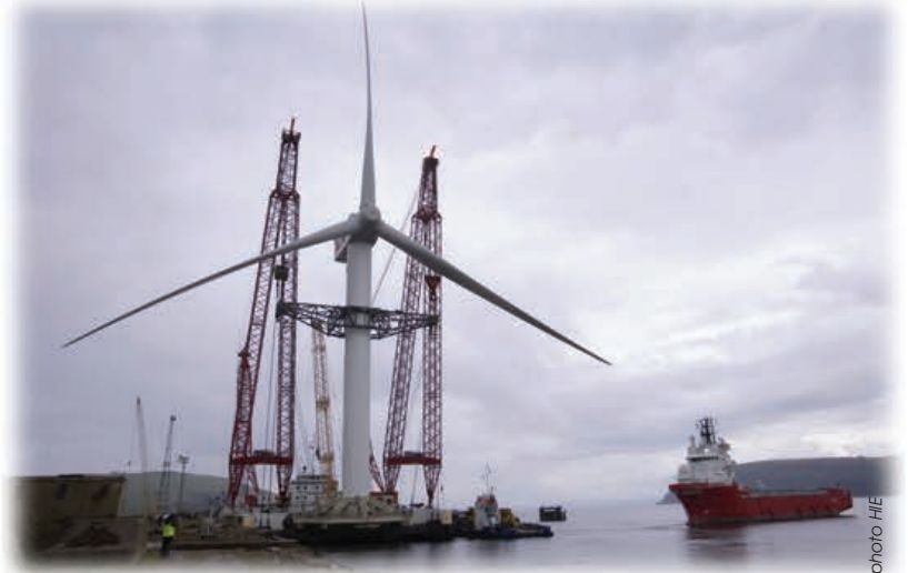
The first Talisman Energy offshore wind turbine leaving the Cromarty Firth by barge on its way to the Beatrice Oil Field in the Moray Firth.
